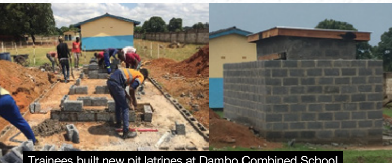
Trainees built new pit latrines at Dambo Combined School
