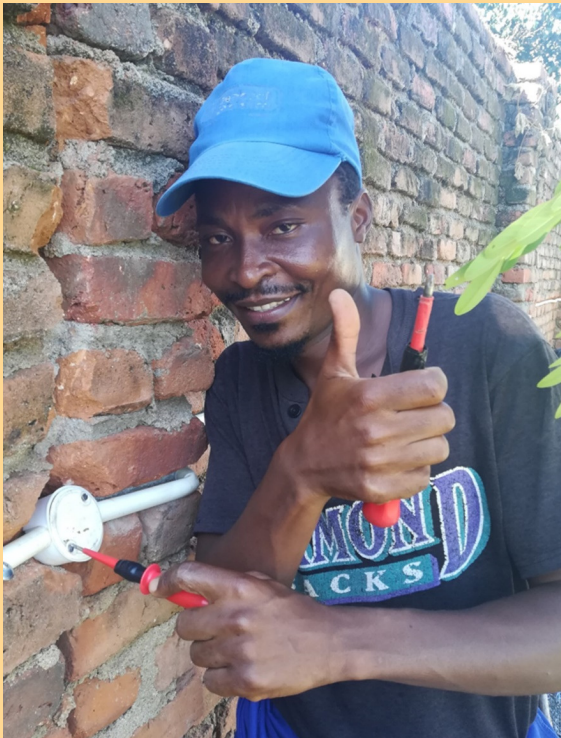
Evance Mteteka set up his own electrical installation business after graduating
